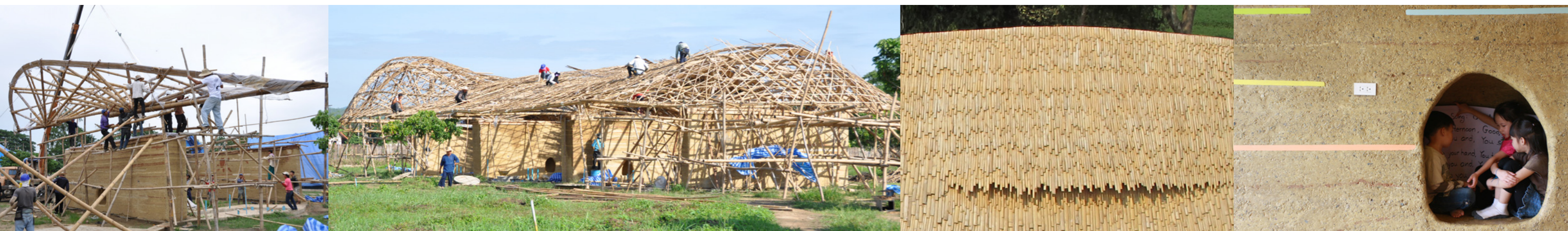
Construction of classroom pavilions
