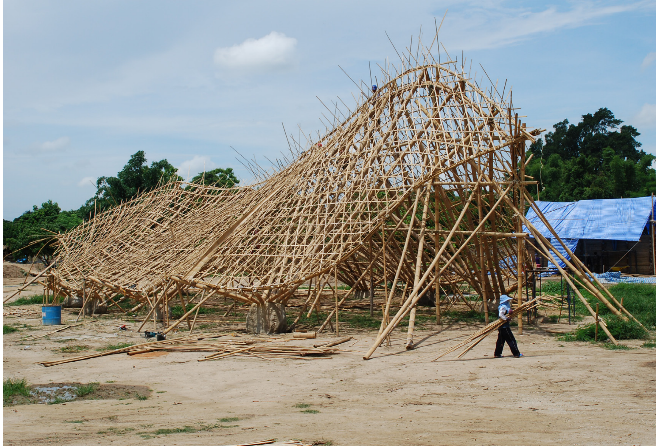
Construction of assembly hall
