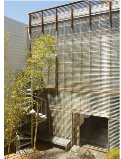
RECYCLED PLASTIC FACADE, DAY
