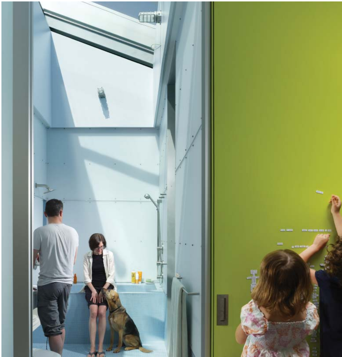
OPERABLE SKYLIGHT - PASSIVE VENTILATION
