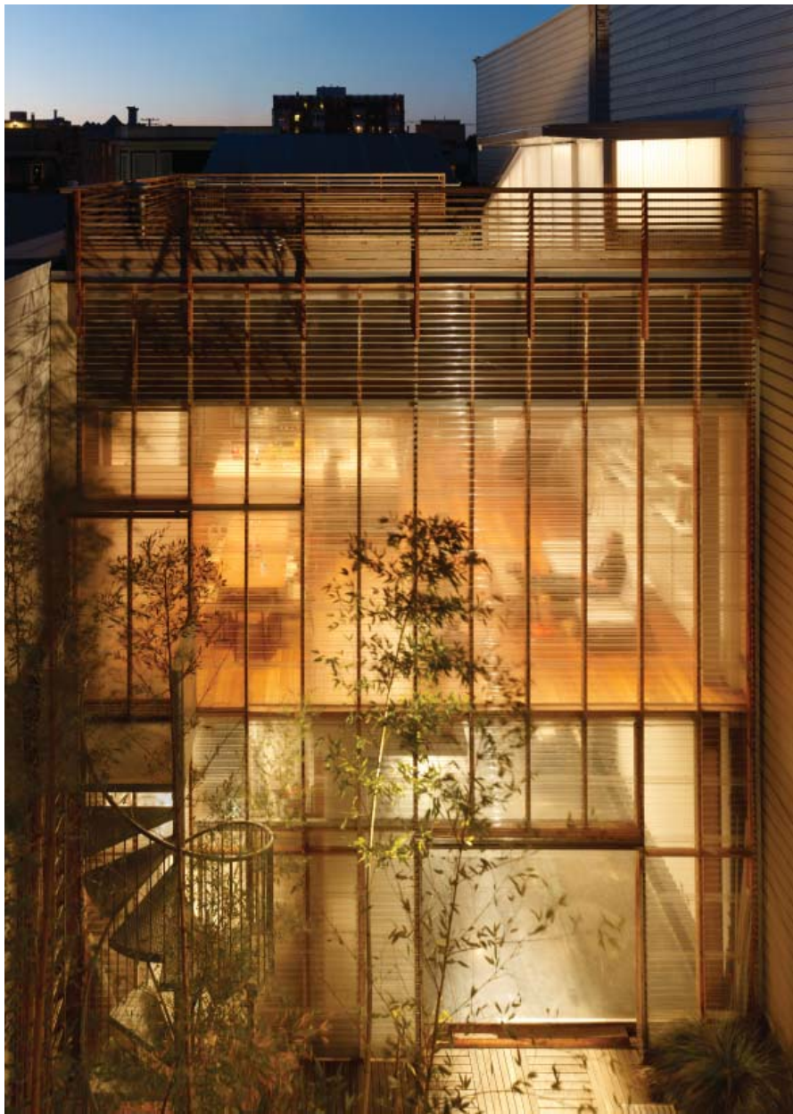
THERMAL PLASTIC FACADE, NIGHT
