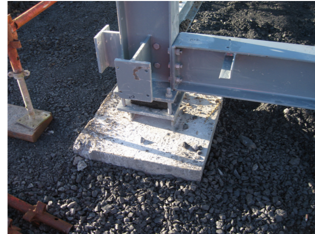
Detail of Thermally broken Steel Frame
