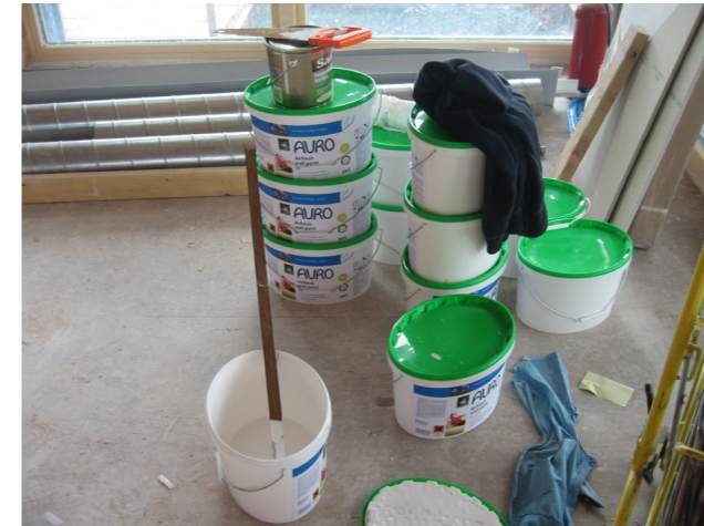
'Fresh Air Paint' used internally on all surfaces.
