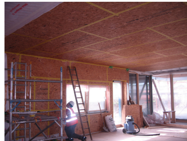
OSB timber sheeting sealed with airtight tape.
