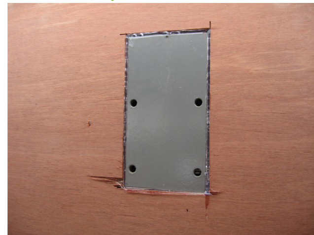
Fixing point from structural frame to exterior.
