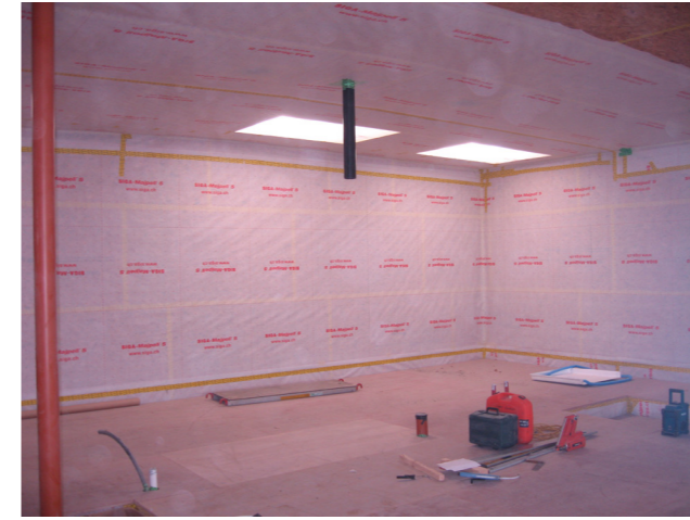
Internal Vapor Membrane on external walls.
