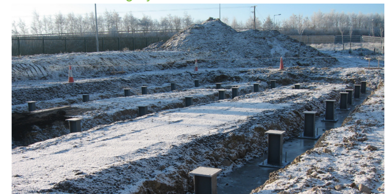
Building separated from cold by thermally broken columns
