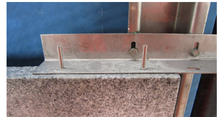
Detail of dry fixed demountable external cladding system for external stone cladding.
