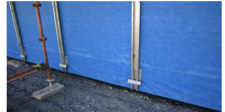
Demountable Fixing System bolted to Structural Steel Frame
