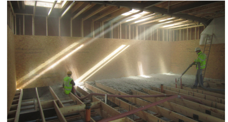
View of building underconstruction showing DfD materials including bolted steel frame, bolte fixed main timber studs, screw fixed timber boarding internally and externally and blown in cellulose insulation from recycled newspapers left on trains.
