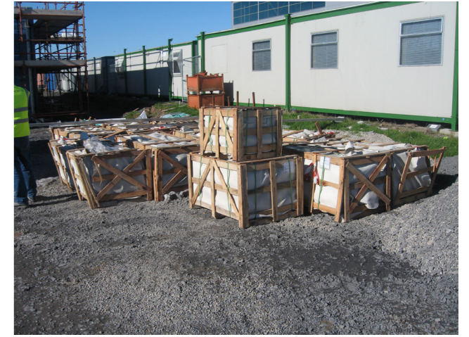
DfD Stone panels as delivered to site.
