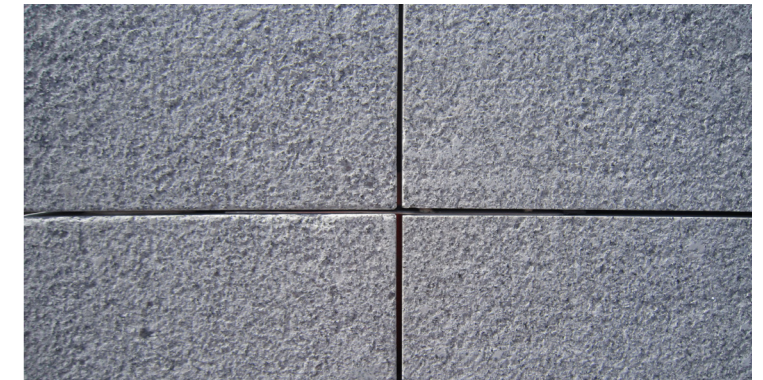
Open Jointed Demountable Granite Cladding ideal for DfD
