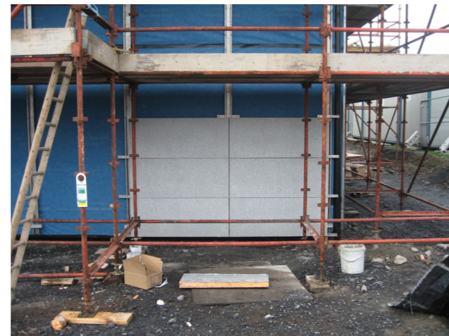
Steel Frame and Stone clad but 95% wood products!
