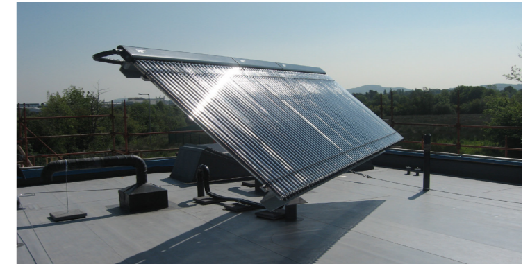
Solar Thermal Collector provides 70% of annual hot water
