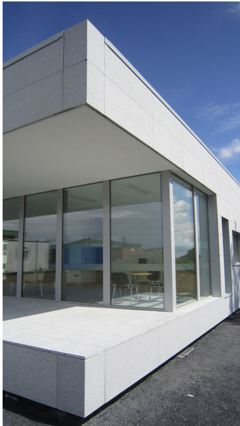
Photograph Showing deep solar control overhang
