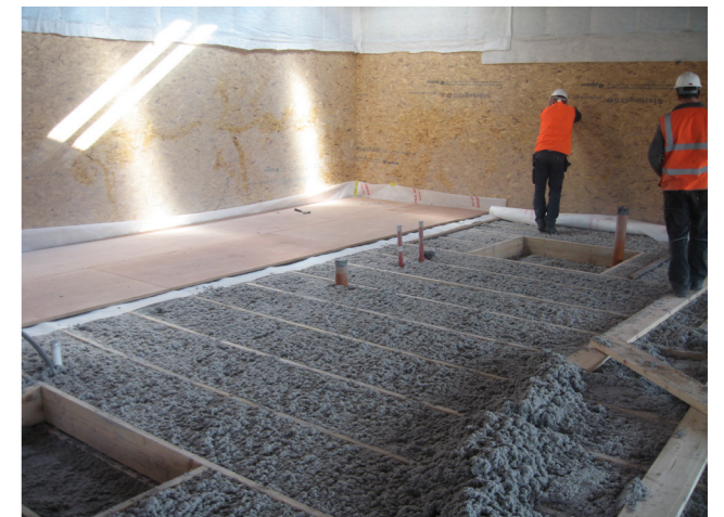
Steel Frame and Stone clad but 95% wood products!
