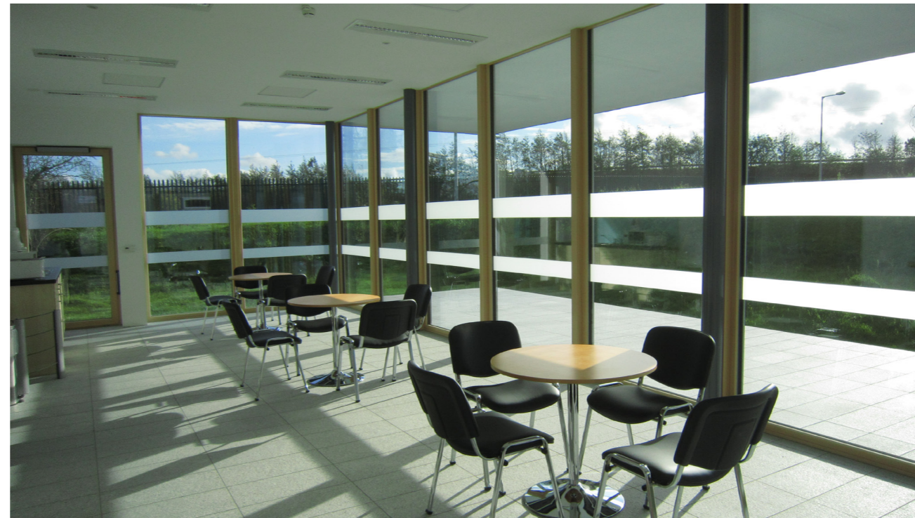
Photograph Showing stone floor used as a heat sink to soak up sun's energy in winter.
