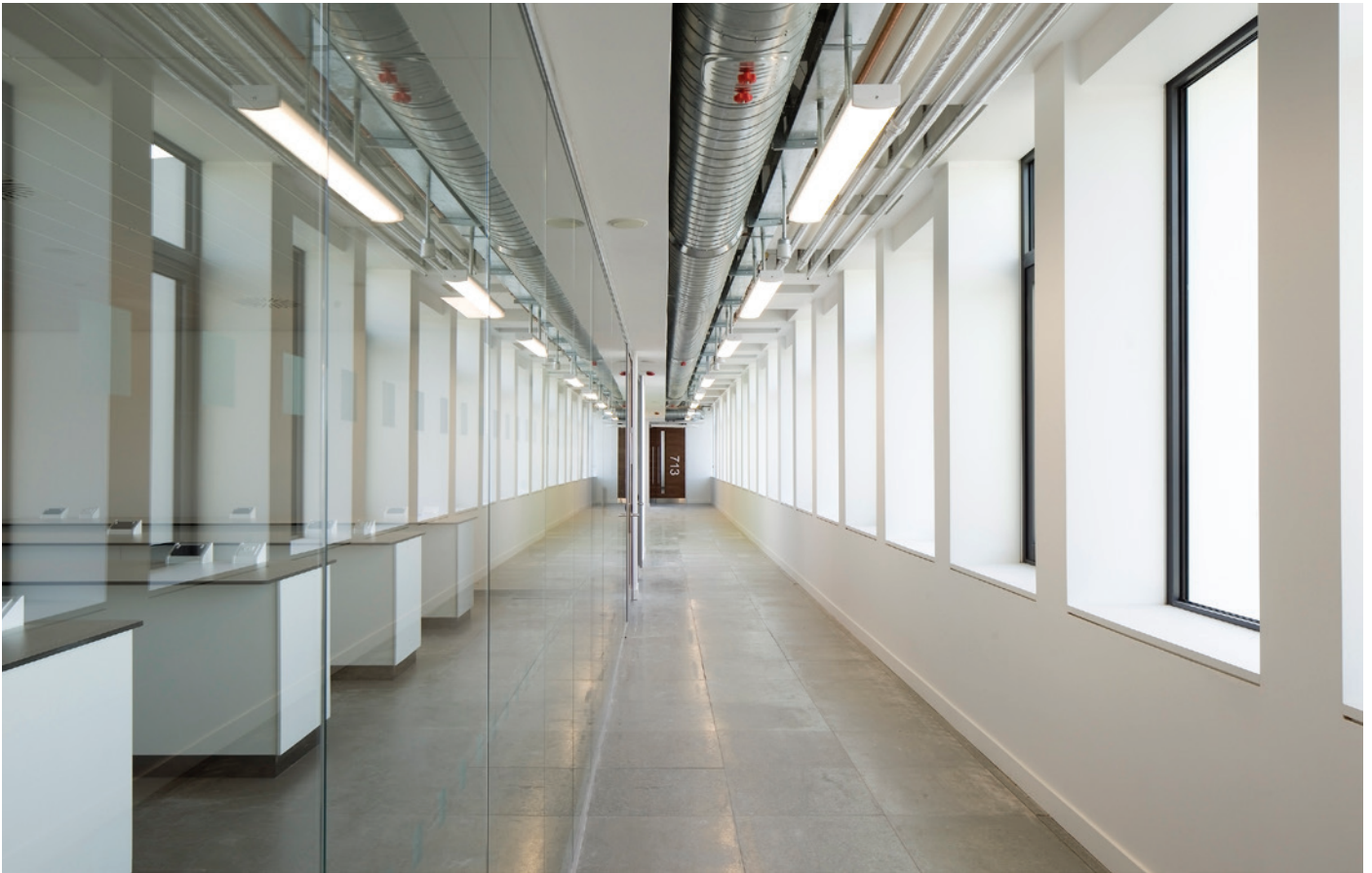
Photo of 7th floor solar corridor
