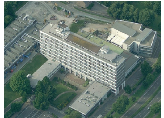
Aerial view of the building
