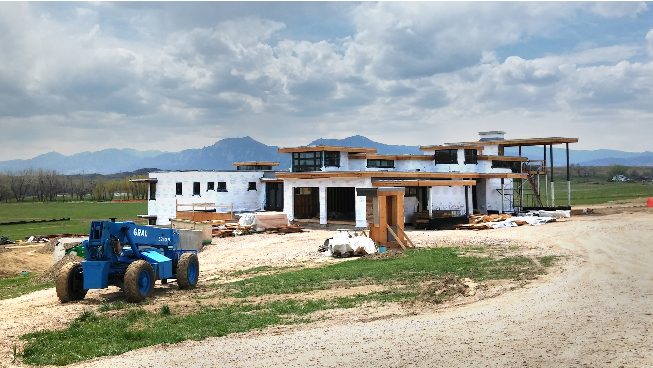
Current Progress - May 2014
