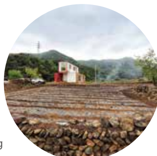
Assembly and Placing
